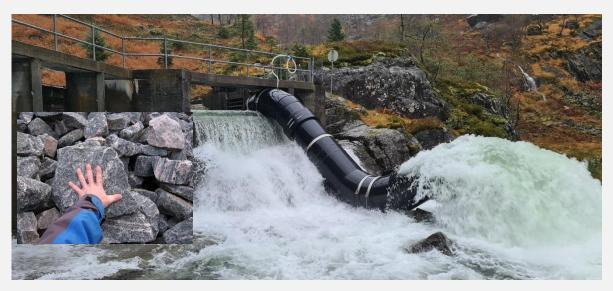
1000 mm diameter boulder excluder at Ulvik Power Plant discharging 5 m<sup>3</sup>/s and sucking away any rocks in front of intake
