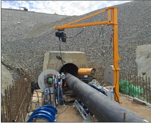
Installation of outlet pipe
