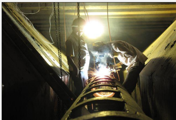
Installation of SediCon Sluicers
