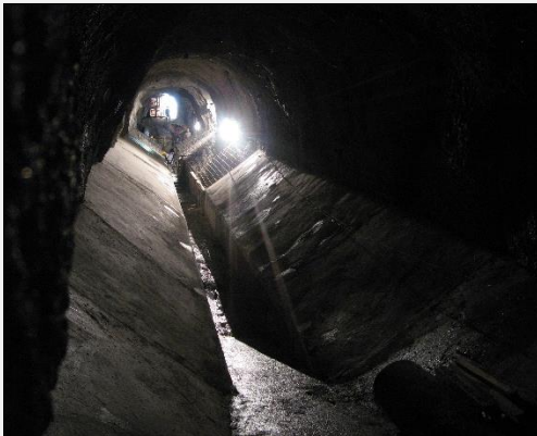
Tunnel desander during construction
