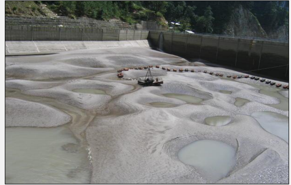
Removed sediment deposits
