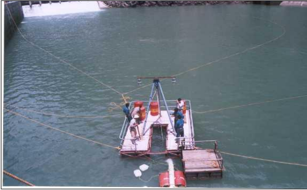
SediCon Dredge at Malana HPP
