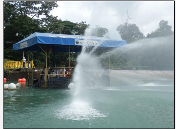
Powerful water jetting disintegrates sediments
