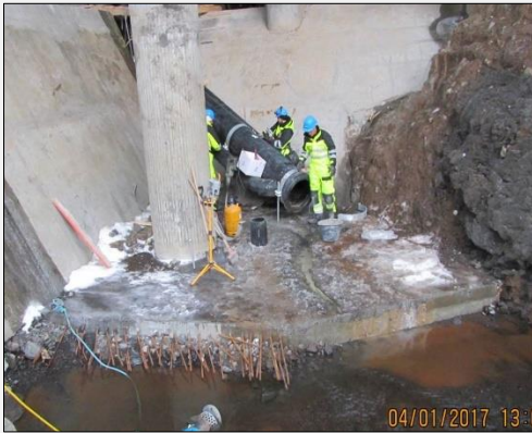
Installation of Gravel Excluder
