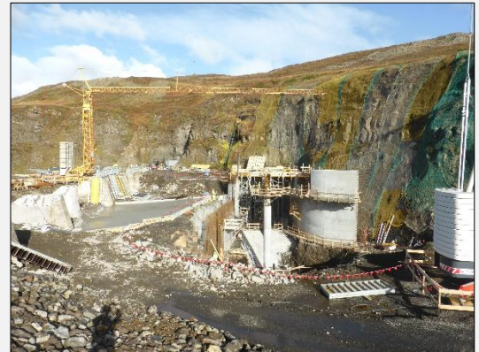
Construction in progress
