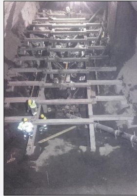
SediCon Sluicer in the desander
