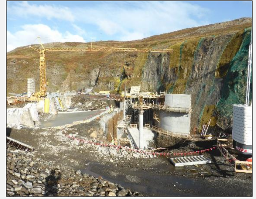
Construction in progress
