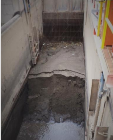
Sediments during maintenance stop
