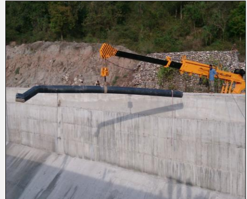
Installation of HDPE pipe
